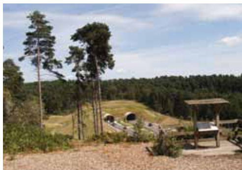
A view of the A3 Tunnel - South portal
